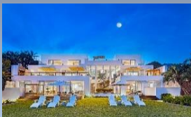
THE WHITE HOUSE BOUTIQUE VILLA
